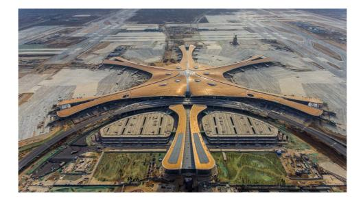
Complex technological solutions were employed in the airport's construction. Thousands of dampening elements are built into the building's steel base. They create a layer that cushions and compensates for the vibrations from airplanes taking off and trains rushing by at high speed.
