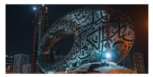
The torus shape is supported by 890 stainless-steel-clad glass fibre reinforced plastic (GFRP) panels that form the seamless silvery façade. The thousands of interlocking steel triangles were produced by 3D printers. Cut out of the panels are phrases of poetry, which are a real differentiator and also act as the museum's windows. The poetry was written by Sheikh Mohammed Bin Rashid Al Maktoum, Dubai's ruler. After dark, the cursive script will be illuminated by 14 kilometres of LED lighting.
