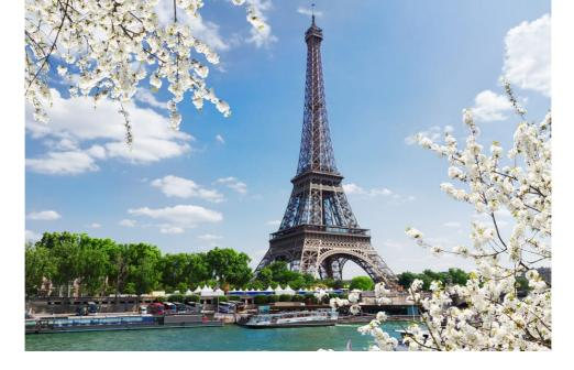
It is estimated that the mass of a similar structure could be reduced by 4,000 tonnes. This would make a modern Eiffel Tower weigh about 3,300 tonnes while maintaining its full strength. In addition, the rivets would probably be replaced by electric welding.
