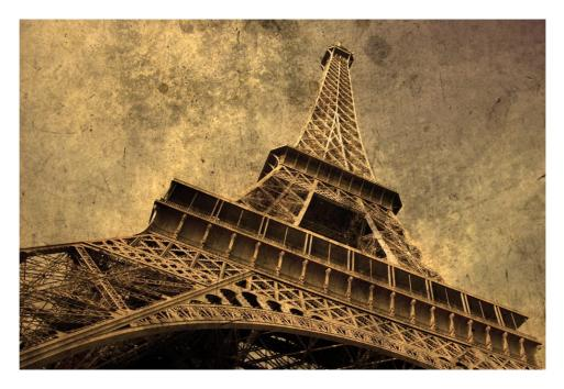
To account for the impact of wind on what was then the tallest structure in the world – it is much stronger at that height than closer to the ground – the project's designers made changes that affected the aesthetics.
