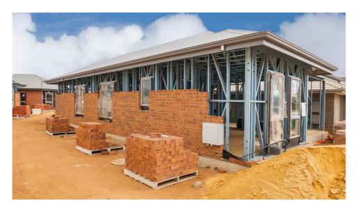
Detailed calculations show that significant savings in terms of both materials and construction technology can be achieved when building a house out of steel. For example, lighter house structures impose less stringent requirements for foundations.
