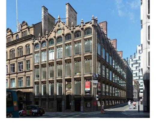
In 1864, this method was tested in Liverpool during the construction of an office building called the **Oriel Chambers**. Its distinguishing feature was a steel framework that supported a glass wall. Today, the Oriel Chambers is considered one of the most outstanding architectural masterpieces of its time. In the late 19th century, though, the building's design met with mixed responses. For example, the UK's oldest business magazine, The Builder (renamed Building in 1966), called it "ludicrous".
