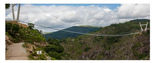
The companies Itecons and Conduril collaborated with the Portuguese National Civil Engineering Laboratory to construct the bridge. The structure of the steel suspension bridge consists of two concrete supports with cables stretched between them and 127 suspended steel sections. During the design and testing of the structure, particular attention was paid to the effect of weather and wind on the bridge. The research included wind tunnel testing and took several months.
