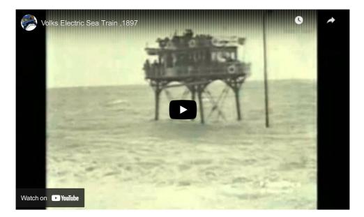
But due to its slow speed, the risk of overturning from the strong waves during rising tides and the difficulties with the construction of wave-breakers, this iron daddy longlegs ran for only five years, from 1896 to 1901. Today, only stone struts, which are visible at low tide, remain as a reminder.
