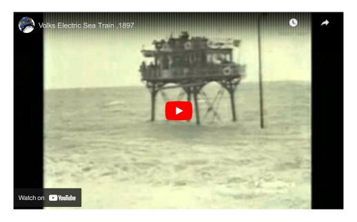
But due to its slow speed, the risk of overturning from the strong waves during rising tides and the difficulties with the construction of wave-breakers, this iron daddy longlegs ran for only five years, from 1896 to 1901. Today, only stone struts, which are visible at low tide, remain as a reminder.
