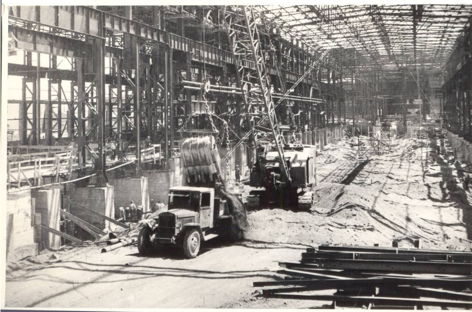
Steel mill construction
