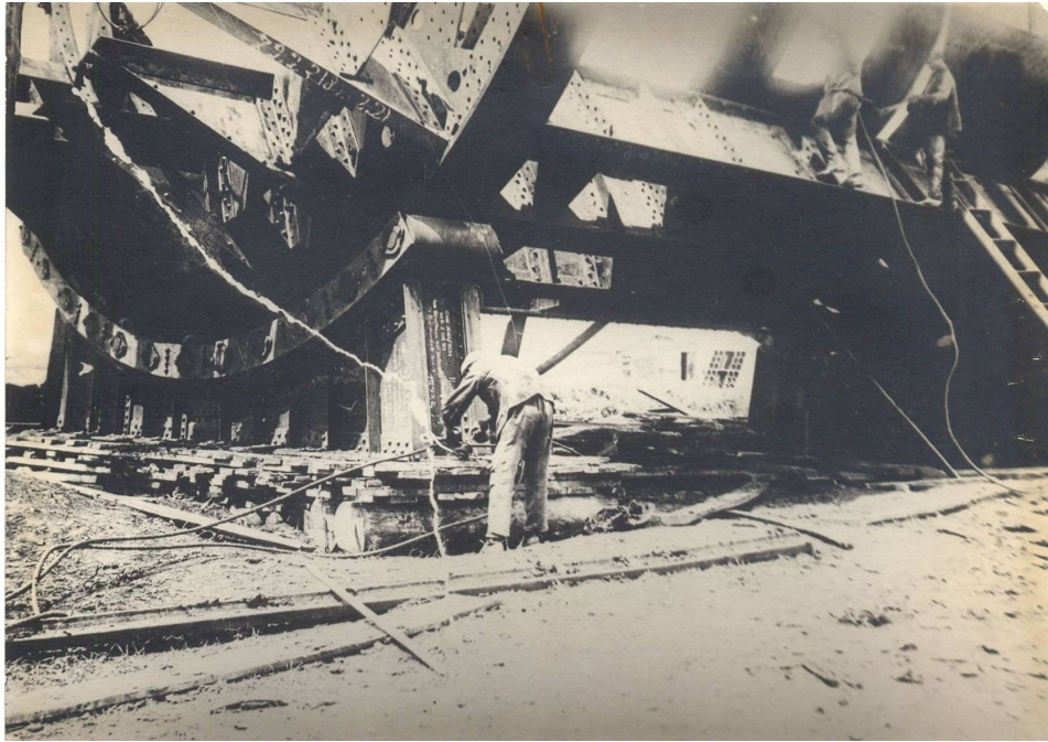
Assembly of the open-hearth furnace in 1935.
