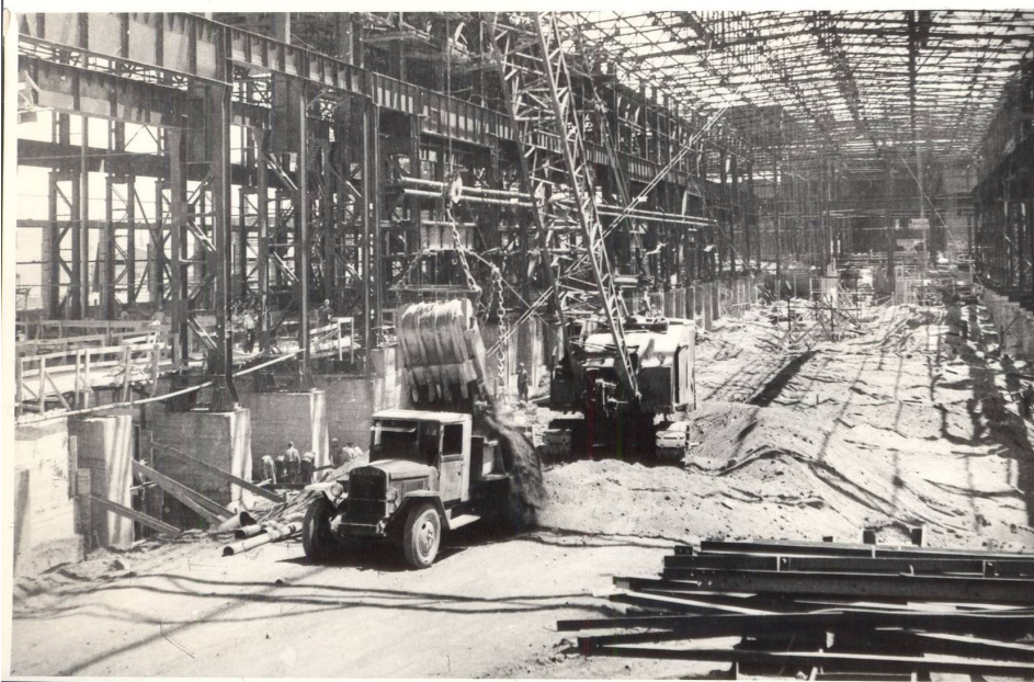
Steel mill construction
