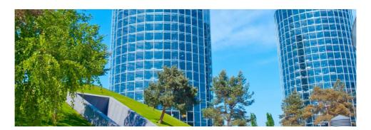
In fact, they are used as a very efficient VW car warehouse, where cars are transported by conveyor belt straight from the plant without having driven even a single kilometre. From the customer centre, any customer can collect their brand-new car with the odometer still reading '0'.
