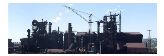
Metinvest modernises the blast furnace facilities as part of its Technological Strategy 2030 that includes a range of environmental projects. Major overhaul will make BF No.6 more efficient, lower production costs, and decrease dust emissions by 55%. All Azovstal's blast furnaces will feature a pulverised coal injection (PCI) system upon construction of the PCI plant at BF No. 3.
