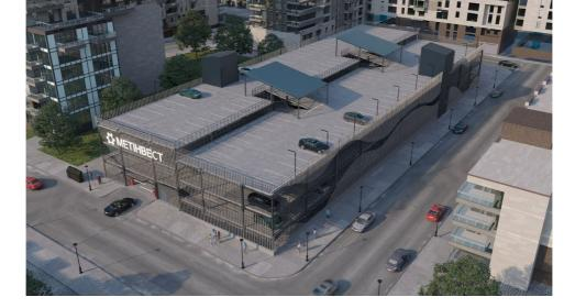
The car park support structures include welded steel beams and columns made of plates, which reduces the building's metal intensity and construction costs. The design provides for reinforced concrete floor slabs with leave-in-place formwork using corrugated sheets.
